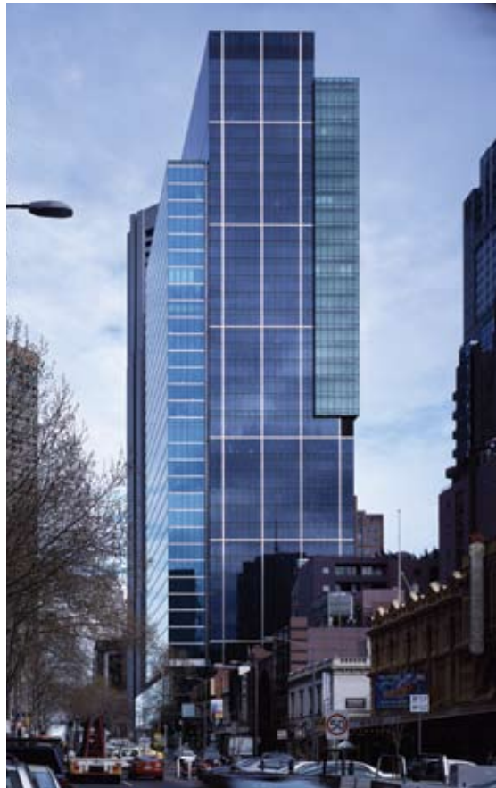
Southern Cross East Tower, Melbourne (Architect: Woods Bagot)
